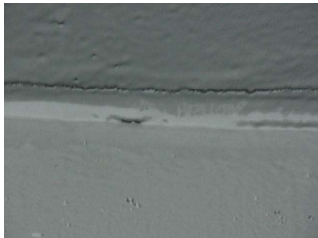
Figure 4: Improper spray technique and resulting “shadows” / “cracks”
