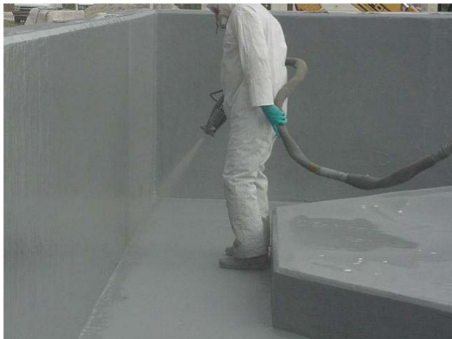
Figure 4: Improper spray technique and resulting “shadows” / “cracks”
