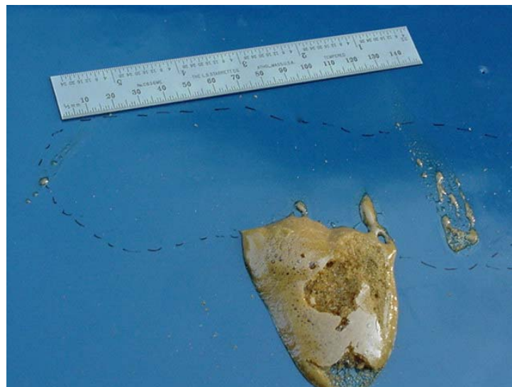
Figure 12: Application over un-cured polyurethane primer Coupled with primer oozing through a pinhole
