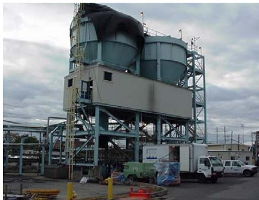
The application procedure called for abrasive blasting of the steel bin interiors to remove the epoxy system. This proved very difficult and air chipper / hammers had to be used to initially remove the 2-coats of flake filled epoxy. The area was then re-blasted to remove the corrosion and provide for a 3-4 mil profile. This was a complete confined space application so all the appropriate OSHA PPE was required.
