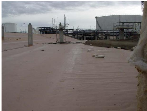
Figure 16: Coated Geotextile Application, CANADA
