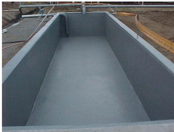
Figure 15: Concrete tank lining
