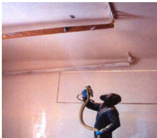
Figure 8: Wall & Ceiling Coating Application
