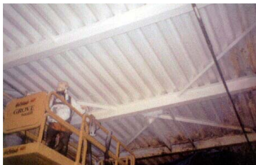
Figure 9: Ceiling Coating over Asbestos
